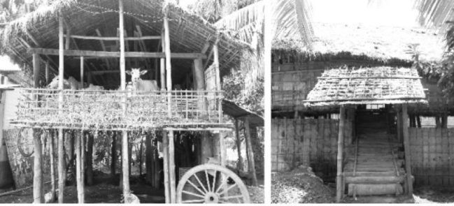
Multi-storied cattle shed (Photo –Jayanta Kr. Sarama )
